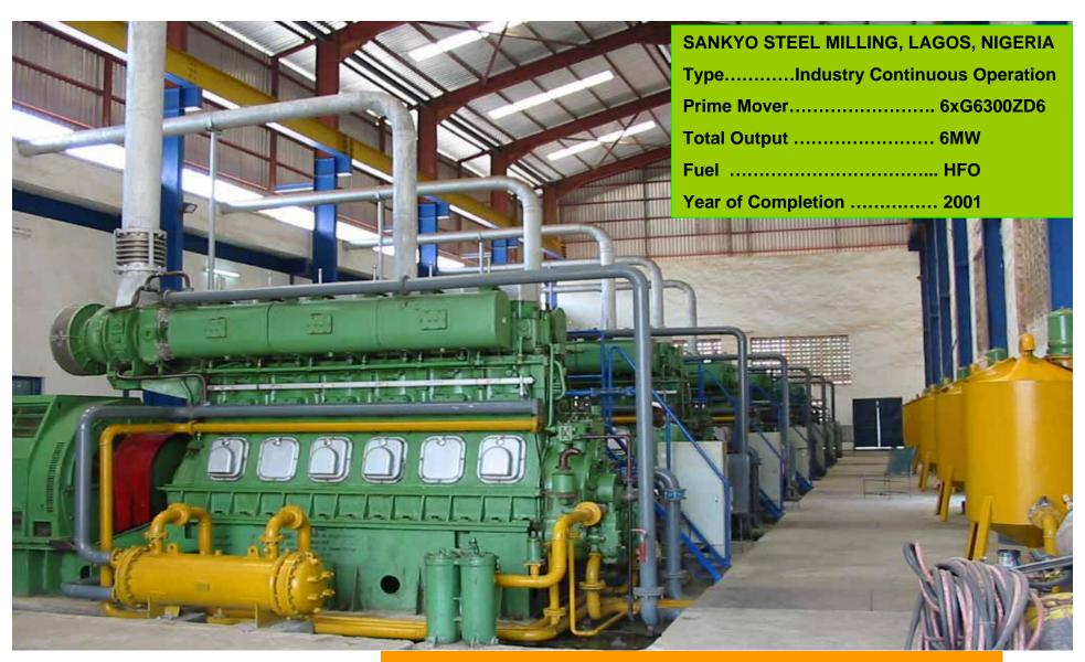
3.3kV supply to steel milling factory
